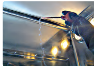
Unidirectional Air Flow Verification (Smoke pattern test)
